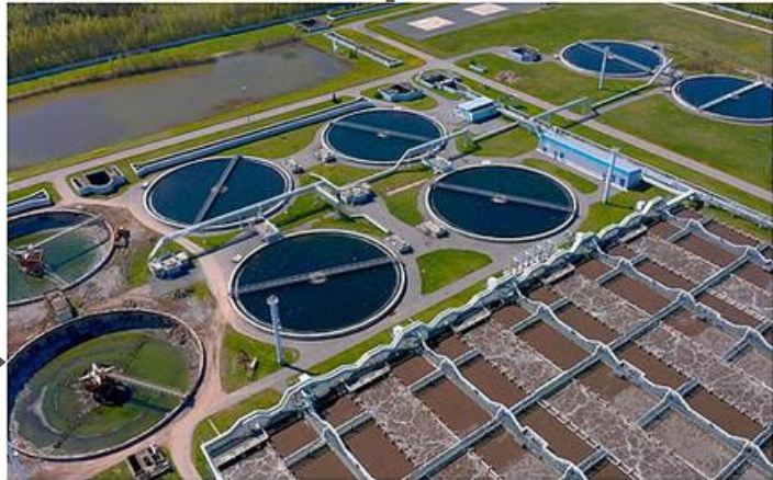
Sewage Treatment Plant
