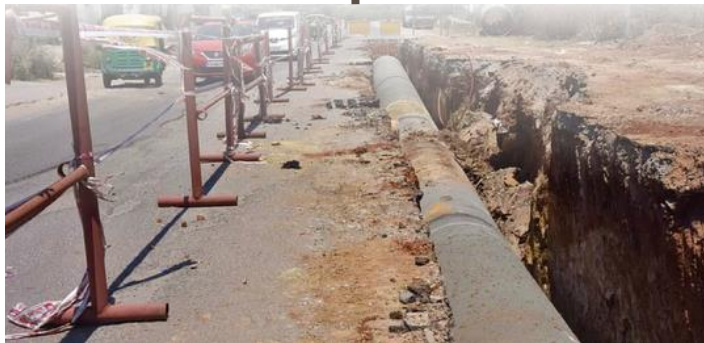
Pumping TWW via Pipeline
