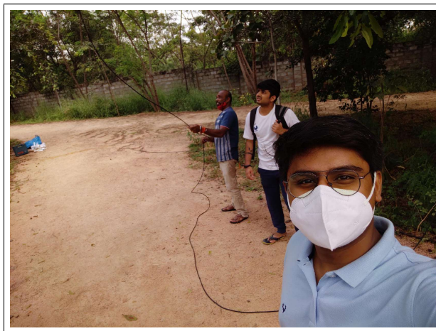
Figure 5.1: Providing power connection in Botanical garden
